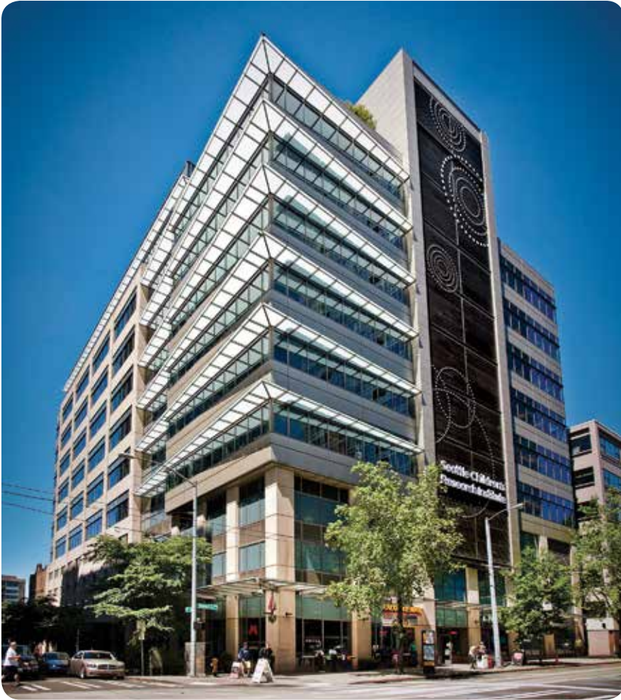
Seattle Children's Research Institute's Jack R. MacDonald Building at 9th and Stewart in downtown Seattle.
